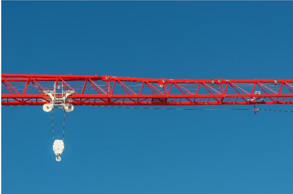
The transition of the jib sections in 4-chord design to the jib sections in 3-chord design. On the right, the hoist rope support, which reduces the rope slack from the standard 10 meters to only 1.5 meters.
