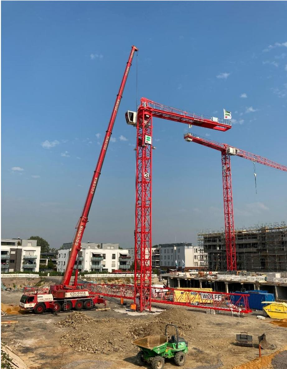
Assembly and dismantling are planned in detail beforehand. This photo shows the raised ramp for the mobile crane and truck in the construction pit.
