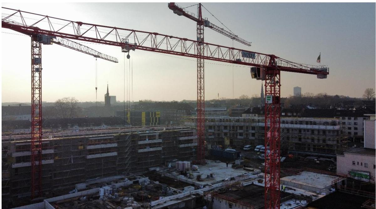
The low assembly height of the flat top WOLFF Clear crane keeps the crane concept low and thus profitable. The entire construction site of 15.600 m<sup>2</sup> is covered with only three cranes.
