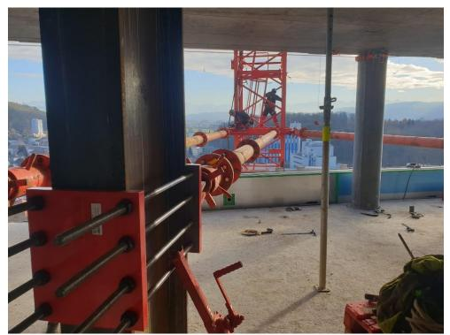
The two tie-ins, which connect the WOLFF 6031.8 Clear to the building, had to be attached to columns inside the building and the facade elements built around them.
