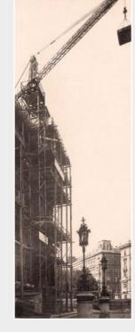
1928 WOLFFKRAN manufactured the first saddle jib tower crane with an electrical trolley.
