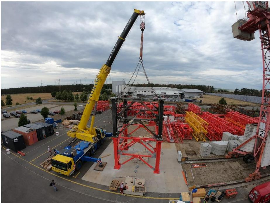
At the end of June, the new tower element was assembled for the first time on the factory premises in Luckau for testing. With external dimensions of 6 x 6 meters, it weighs 28 tons. Heavy equipment is required for its assembly.
