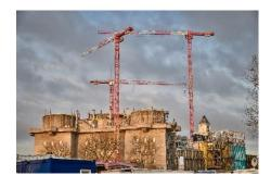
Thanks to their flat-top design, the WOLFF clear cranes can slew 10 meters above one another and the overall crane concept for the Flak Tower project thus kept relatively low.
