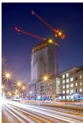
Thanks to the economical assembly concept, the two WOLFF cranes are a mere 47 meters apart and can slew directly one below the other.
