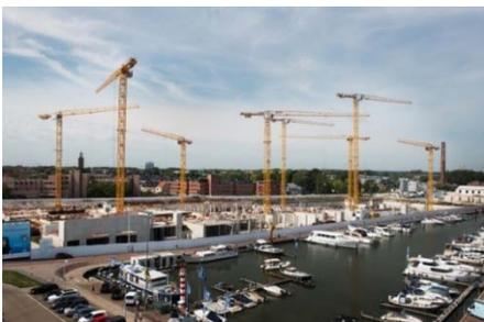
Thanks to precisely coordinated hook heights and jib lengths, the cranes can slew past each other effortlessly while moving building material on the cramped construction site.
