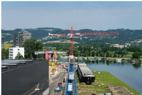
The WOLFF 7532.16 *cross* is used for moving ship dollies and performing maintenance work of the riverboats. Travelling on rails tremendously increases its working radius.
