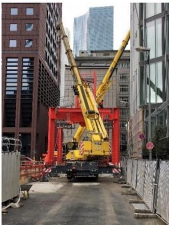
Assembly of the WOLFF Cityportal, with internal dimension of 6.2 x 6.2 meters and a clearance height of 4.5 meters, to ensure the free flow of traffic.
