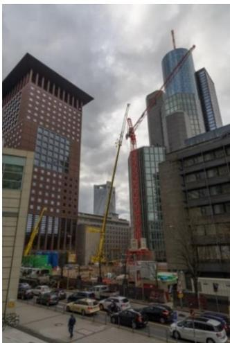
The WOLFF 355 B with its 55-meter jib was assembled to a tower height of 64 meters in just one weekend and will climb to a final tower height of 184 meters during the construction project.
