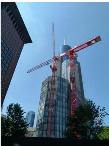
The almost vertical position of the jib and the short counterjib of the WOLFF 355 B luffing crane as well as the flat-top construction of the 6031.8 *clear* make the WOLFFs an ideal choice for large-scale inner-city construction sites.
