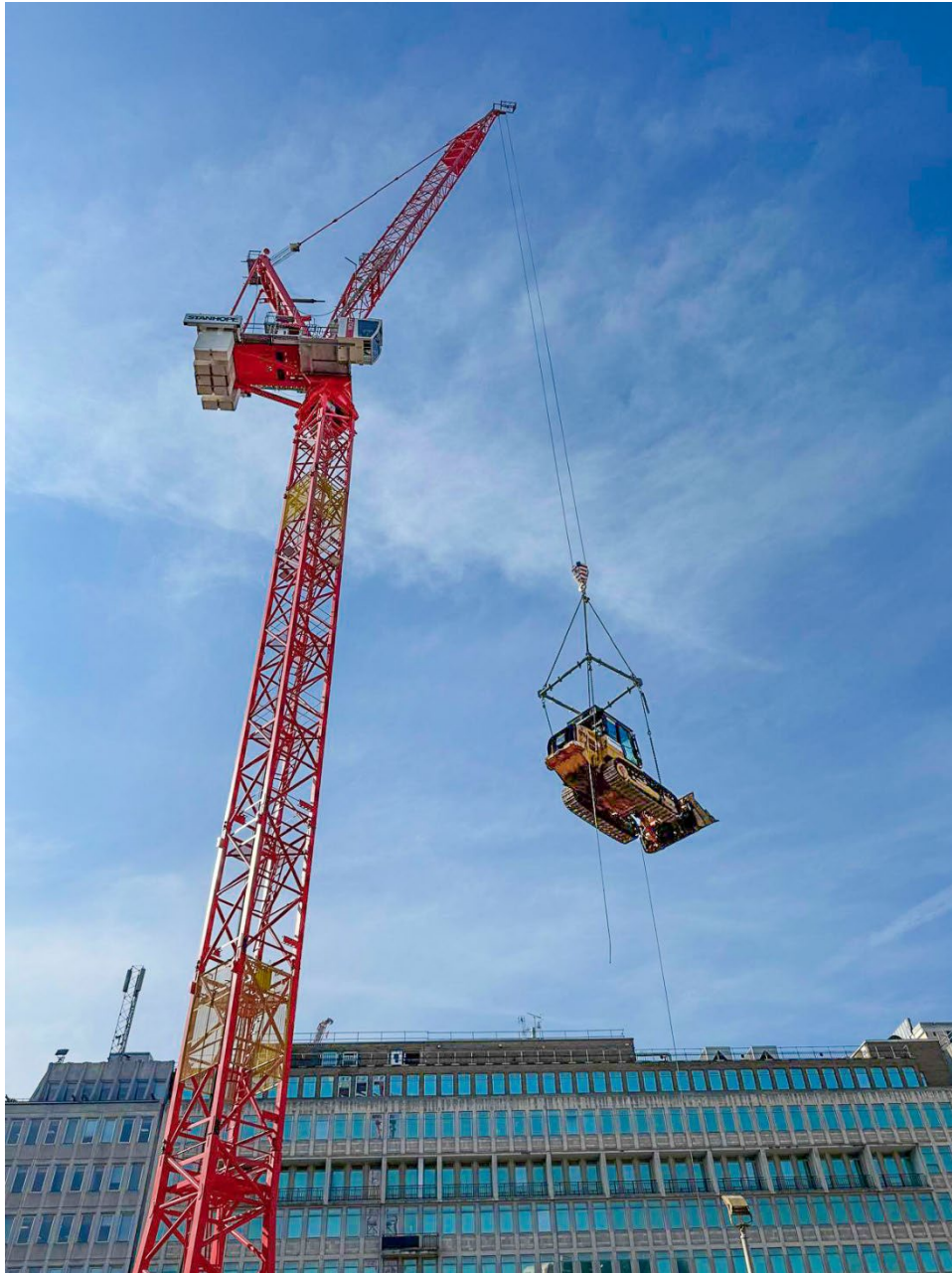
The WOLFF 355 B (TC0) lifting an excavator during the demolition works.
