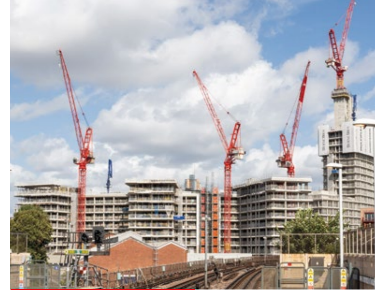
Television Centre Phase 2, London, UK
