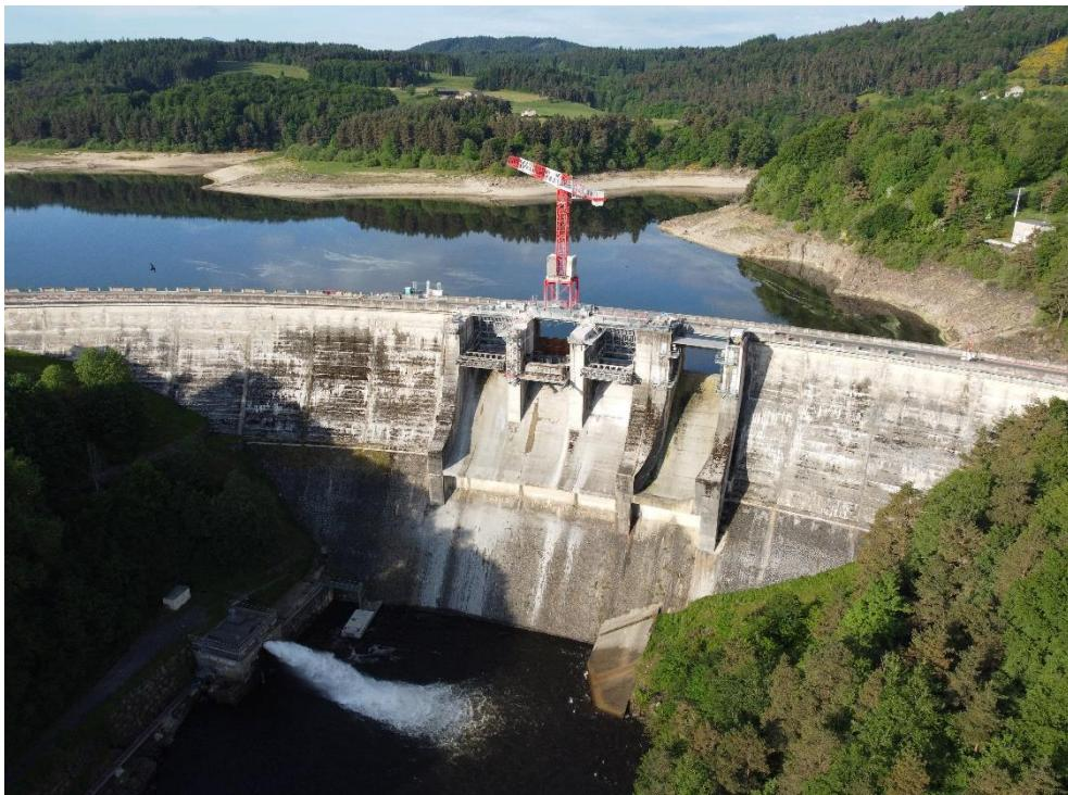
The WOLFF 7534.16 Clear, with a hook height of 20.4 meters, a jib length of 40.0 meters, and a load capacity of 16.0 tons, is replacing the flood gates at the Barrage de Lavalette dam in south-eastern France.
