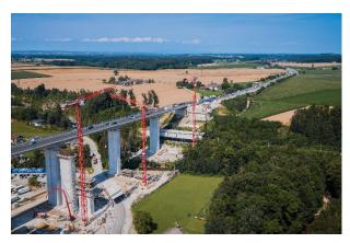
Impressive trio: The WOLFF cranes lifted loads of up to 13 tons during the demolition of the old bridge as well as the construction of the new superstructures and piers.
