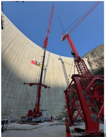
The dismantling took place in two stages. In fall of 2024, the upper, narrower tow-er of the first WOLFF was dismantled. This summer, the lower tower and the com-plete second crane followed. Altogether, the dismantling with a 650-ton mobile crane took around three and a half weeks.
