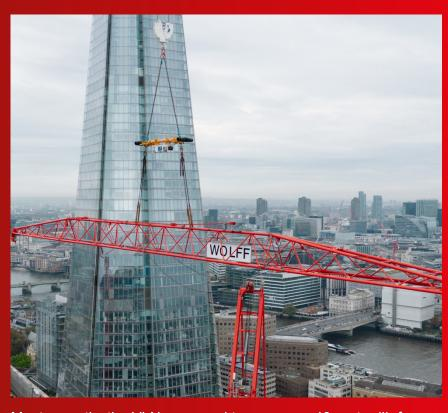
We recently dismantled a crane at the Chapter Living London Bridge project using the Vita Load Navigator (VLN), demonstrating exceptional precision and control. This advanced system detects real-time load movement and adjusts using high-powered fans, preventing spinning and other hazards.
