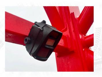
The Crane Climber Detection is the market-leading solution for Construction and Infrastructure projects and Tower Crane protection. The technology has the ability to detect unauthorised individuals attempting to climb the crane or accessing the site. Once a breach is identified, key holders and the police are promptly notified, and a security guard will attend the site for immediate investigation.
