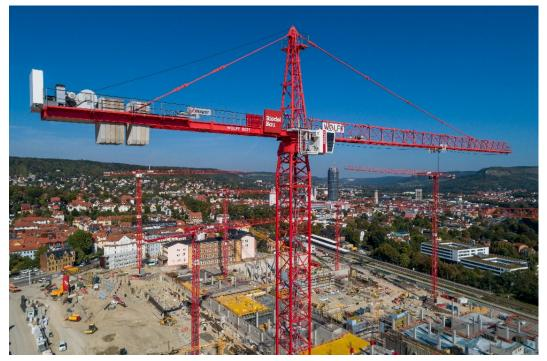
The WOLFF 6071.20 Cross is the powerhouse of the WOLFF pack on the Zeiss construction site. Its job is to lift prefabricated parts weighing up to 22 tons.
