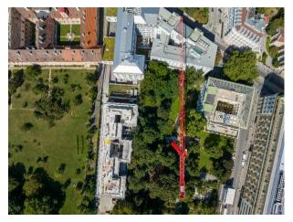
This peak performance allows it to transport any construction materials and prefabricated parts between Prätoriusgasse (in the image on the right) and the construction site, virtually eliminating the need for construction vehicle traffic through the botanical garden, and it was also assembled from Prätoriusgasse.
