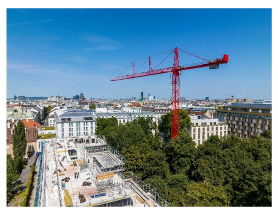
With a 7.0-ton tip load capacity and an 80-meter jib, the WOLFF 8060.25 Cross is currently Austria's most powerful construction crane.
