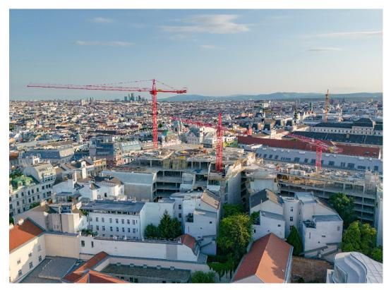
Positioned inside the new building, the WOLFF 7532.16 and the WOLFF 6023.8 cannot be dismantled with a mobile crane. To dismantle the 7532.16 using the WOLFF 8033.16 standing some 60 meters away, its counter jib must be split into two parts while still on the crane, requiring an intricate support solution.
