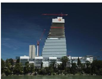
The WOLFF 7532.16 and the WOLFF 180B luffing crane (left) at Roche Building 1. Due to the unusual shape of the building, the initially used WOLFF 6023.8 was replaced by the WOLFF 180 B after a certain height.
