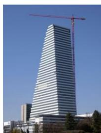
At a 204-meter hook height, the WOLFF 7532.16 was the highest construction crane in Switzerland.
