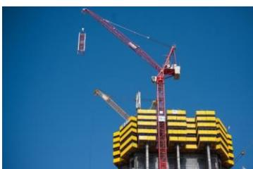
The WOLFF 355 B luffers convinced the customer due to their very high working speeds of up to 185 m/min and a hook path of 920 meters together with significant lifting capacities when compared with the competition for the compact working radius.
