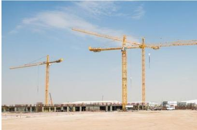
Along with the luffers comes a pack of twelve saddle jib cranes type WOLFF 7532, which are used primarily for moving loads on the ground and for construction of the podium at the base of the tower.
