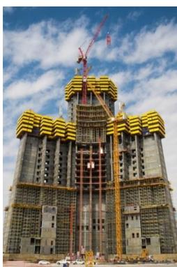
The WOLFF 355 B luffers are raised step by step with the building by means of an internal climbing procedure. One luffer will be replaced several times and will reach a final hook height of around 800 meters.
